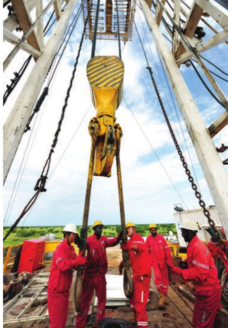
Chinese workers from the Zhongyuan Petroleum Exploration Bureau (ZPEB) of Sinopec and Sudanese workers drill an oil well in South Sudan.
