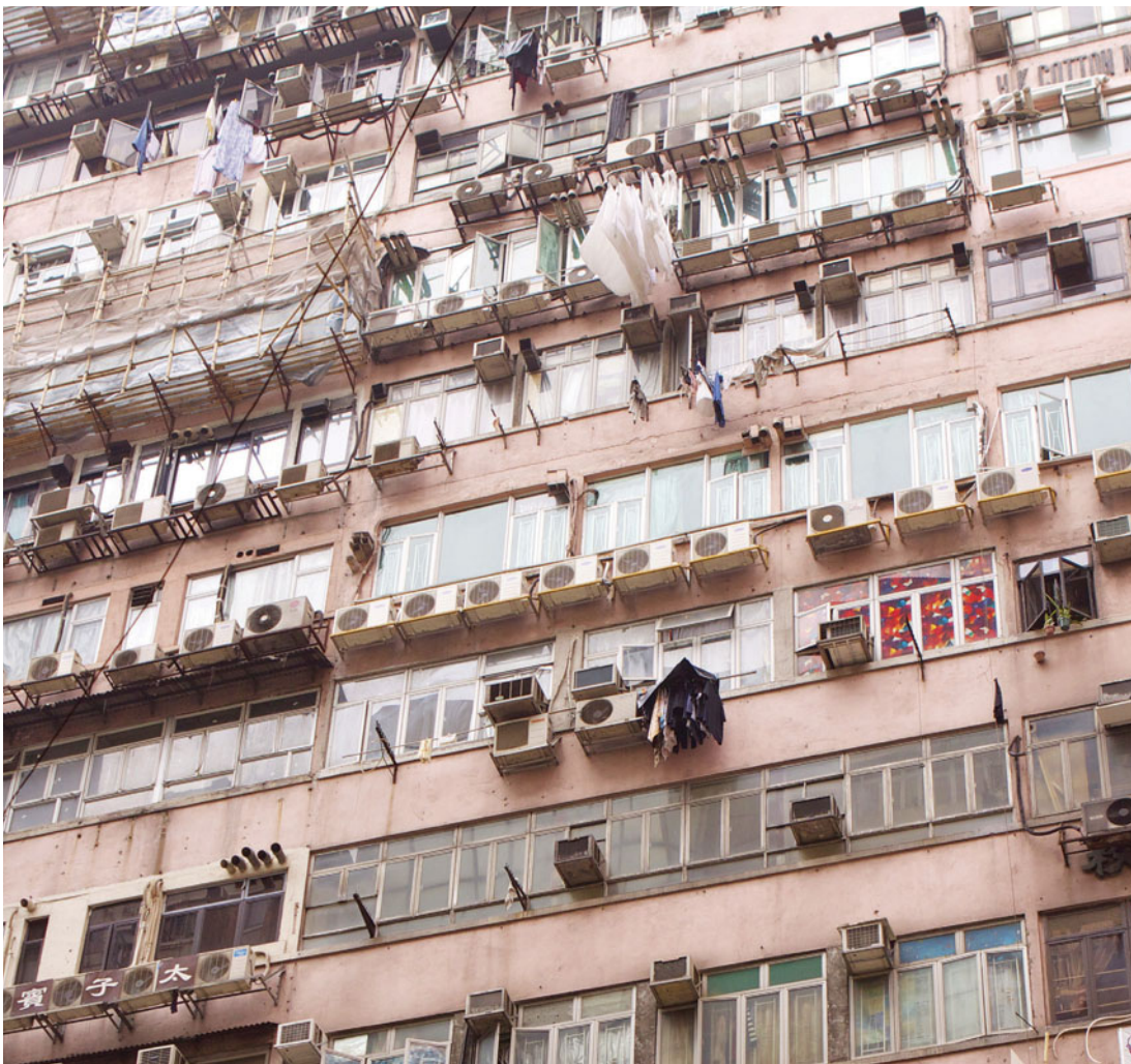
Residential tower with air conditioning units, Hong Kong. Photo by Emma Durnford/Lattitude Stock.
