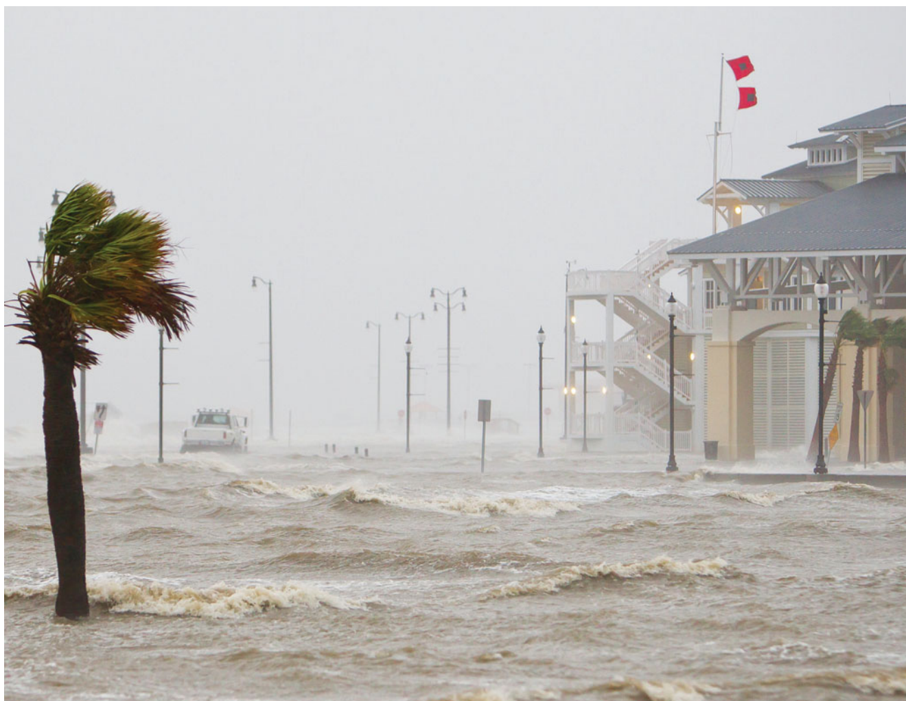
Devastating storm surge during Hurricane Isaac, Gulfport, Mississippi, 2012. Photo by Mike Theiss/National Geographic.
