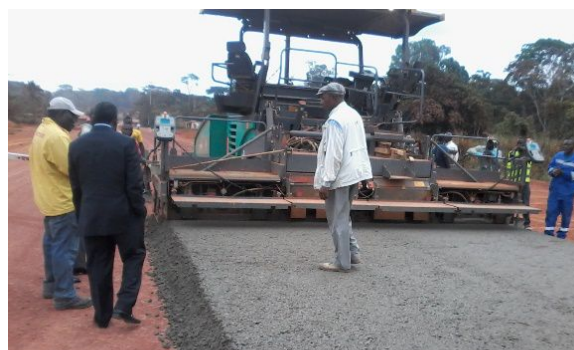
Figure 19 Construction of rural roads in Cameroon
