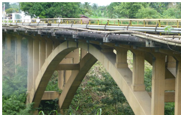
Figure 16 Climate proofing the Roaring Creek Bridge in Belize
