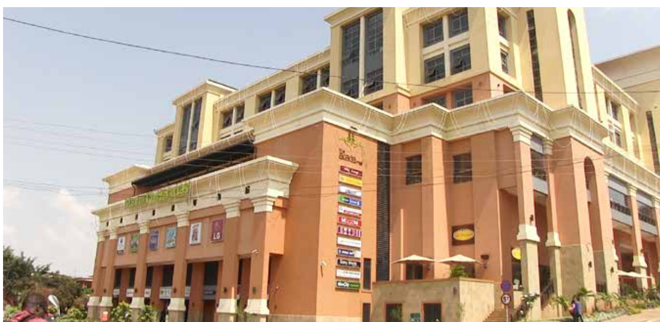
New commercial buildings reshaping the face of Kampala. Digital Media Network Ltd (2015)
