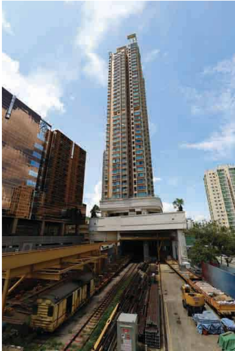
Photo 3.3 Residential towers developed above MTR Corporation's depot at Fo Tan Station
