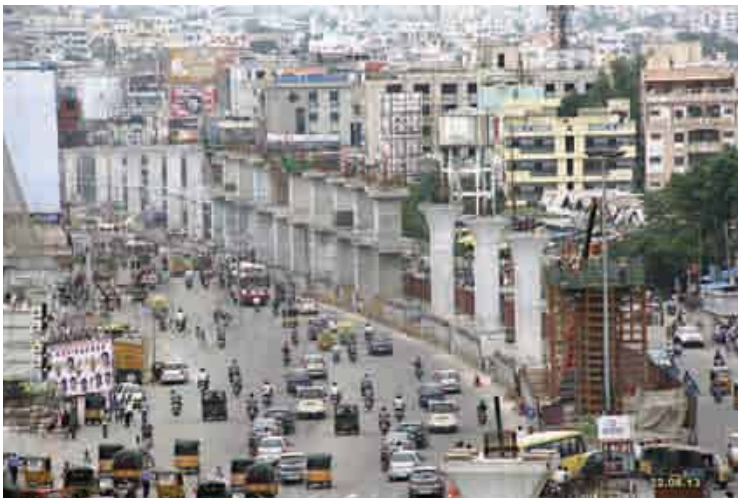
Photo 7.2 Metro construction in progress: Cutting across the built-up areas of Hyderabad
