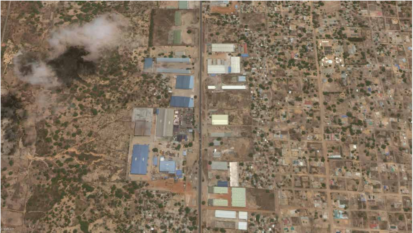
FIGURE 5.7 A residential area (right) is cut off from the main highway by an industrial fence-line in Nacala Porto, Mozambique
