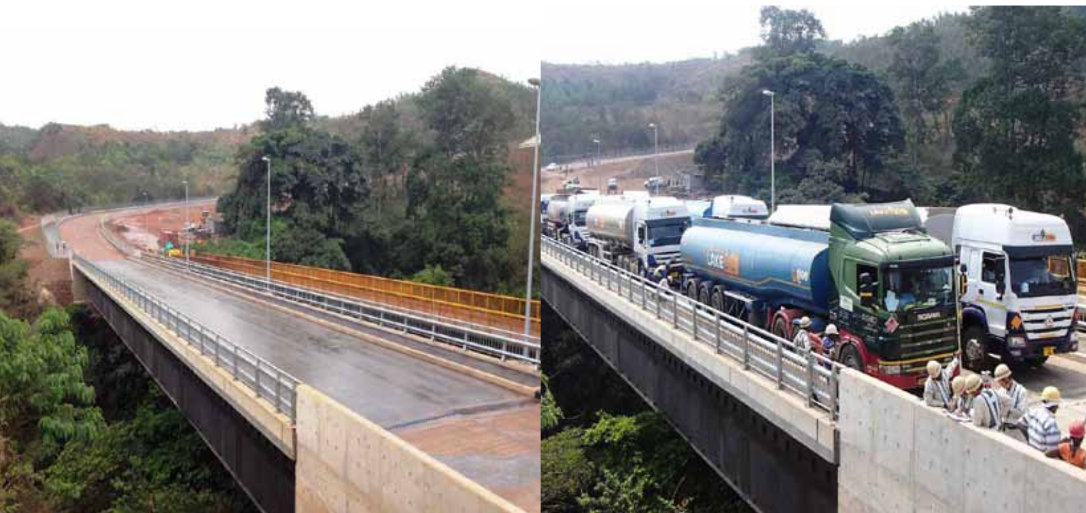
Rusumo International Bridge: Constructed to conform to the EAC Design Codes
